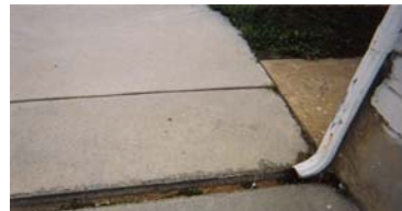
Example of roof drainage across Main Street sidewalk.
